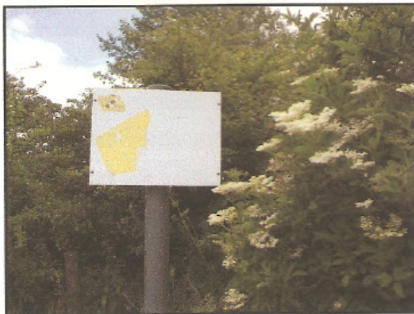
Fig 25 Faded sign at Access 5
