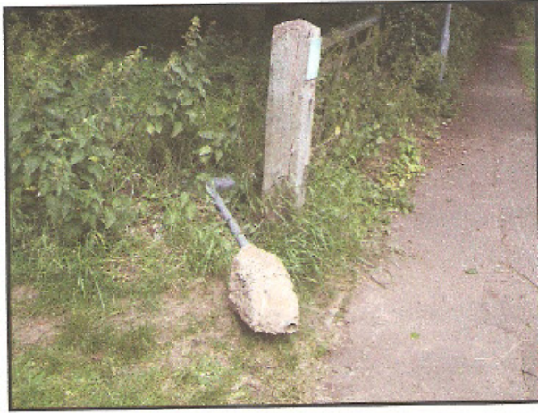
Fig 26 Broken Sign at Access 3
